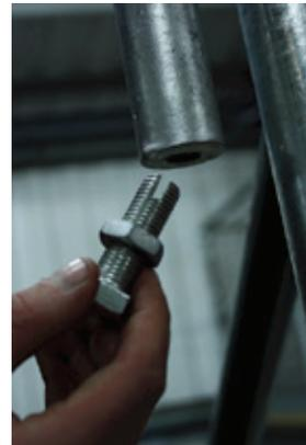
Take the gate and align the top hinge with the upper tang of the spring. (Viewable from the top of the spring housing). Lower the gate into the respective hinge bodies. Set the gate in its CLOSED position between the posts. Turn bolt half turn, to increase spring torsion, in either a clockwise or anti-clockwise direction. This will swing the gate in the direction of choice. The gate can be hung left handed or right handed. Over torsion will damage the internal spring.
