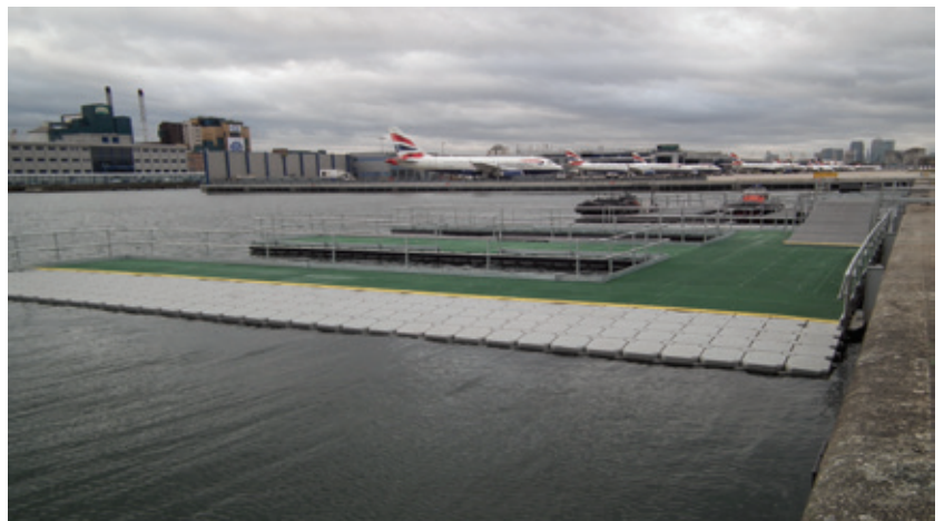
Forginex 11 used at London City Airport
